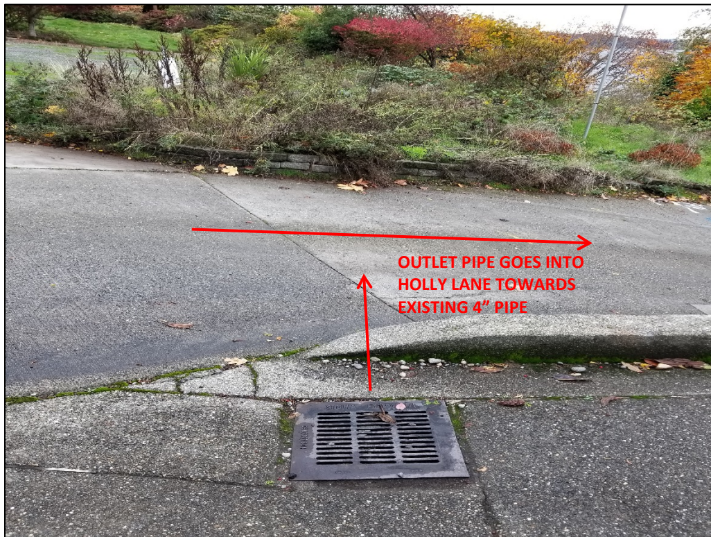
Figure III-5. Area drain in neighbor's driveway across street.
